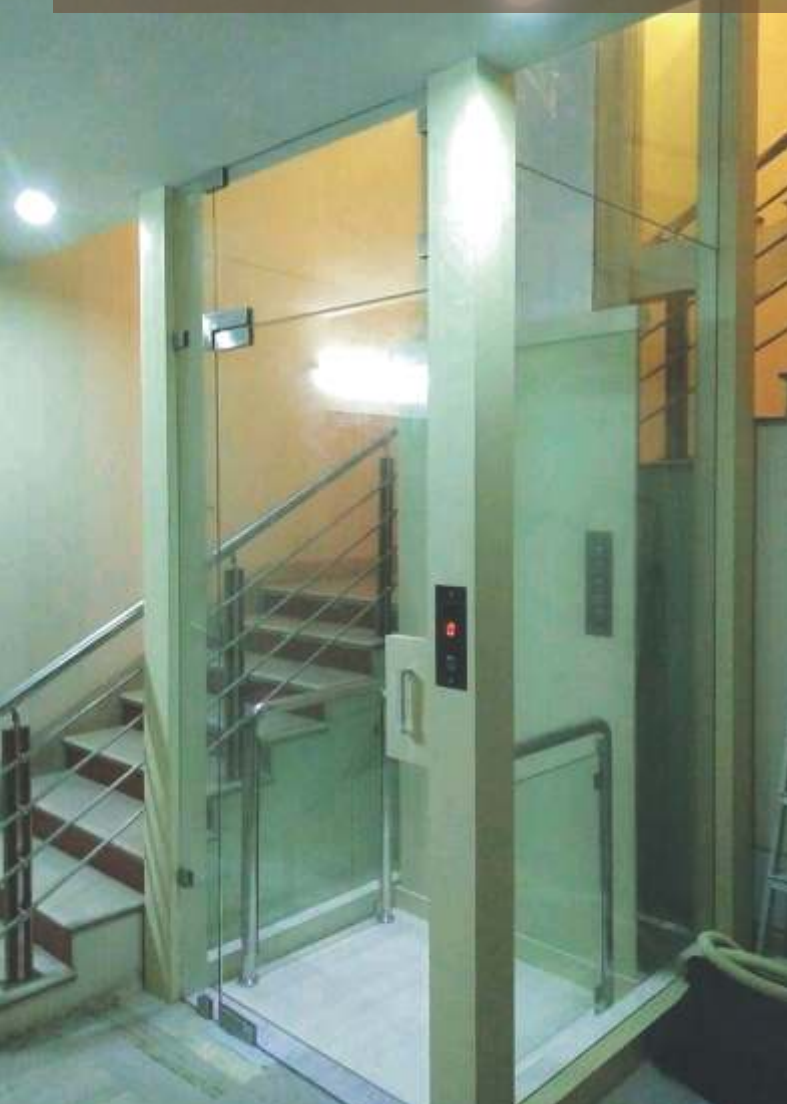
“LEVITATOR®” EXTERNAL INSTALLATION IN BUNGALOW
